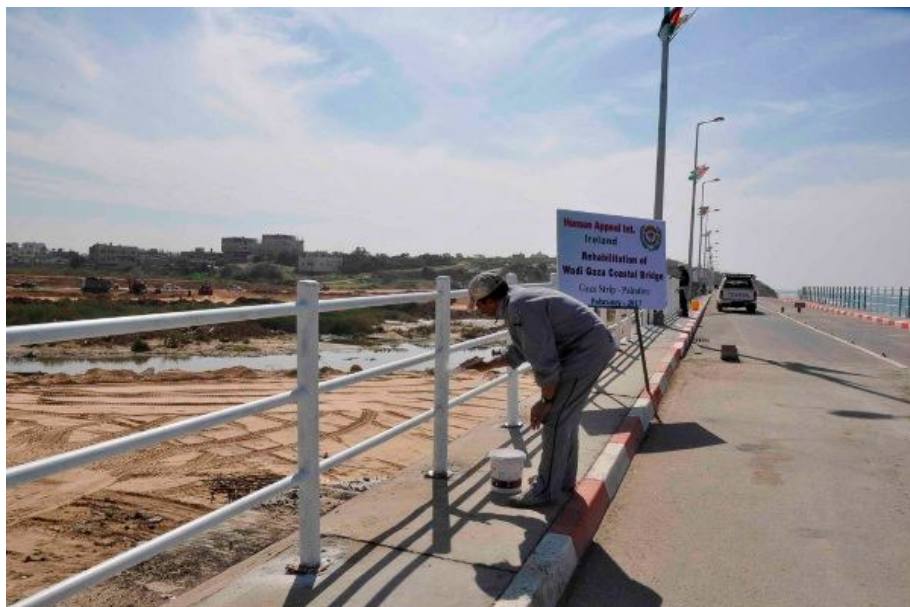
Final touches of repair work on destroyed bridge on Gaza Valley Coastal Road undertaken by HAI.
