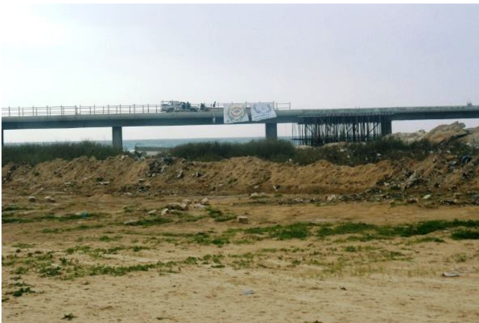
This bridge on Gaza valley was destroyed by Israel.; now being repaired.
