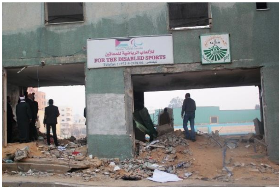
Nothing is safe; not even sport ground for the disabled
