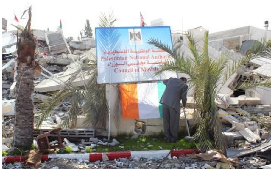
The destroyed Council of Ministers building
