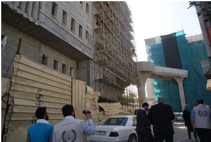
New construction work - Al-Shifa Hospital
